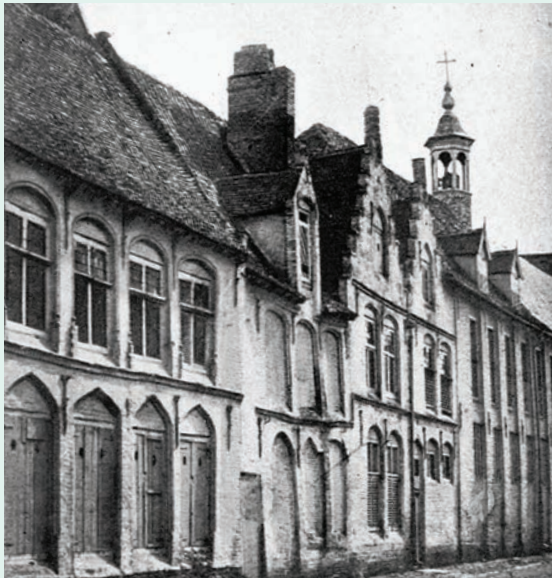
Facade of the old convent on rue Saint-Jacques, Ypres
